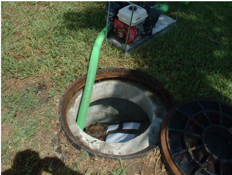
Figure 3-4. Sump Pump-Out Activities for the Stormceptor Unit.
