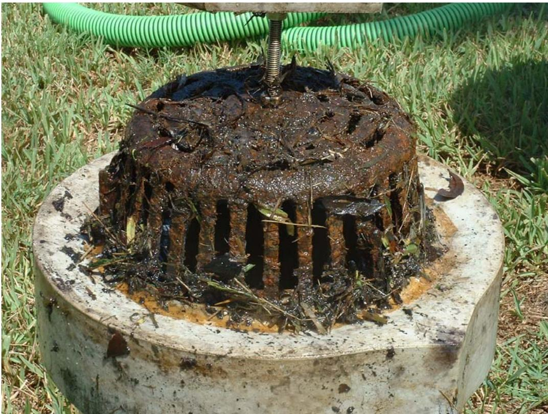
Figure 4-3. Stormceptor Trash Guard Device.
