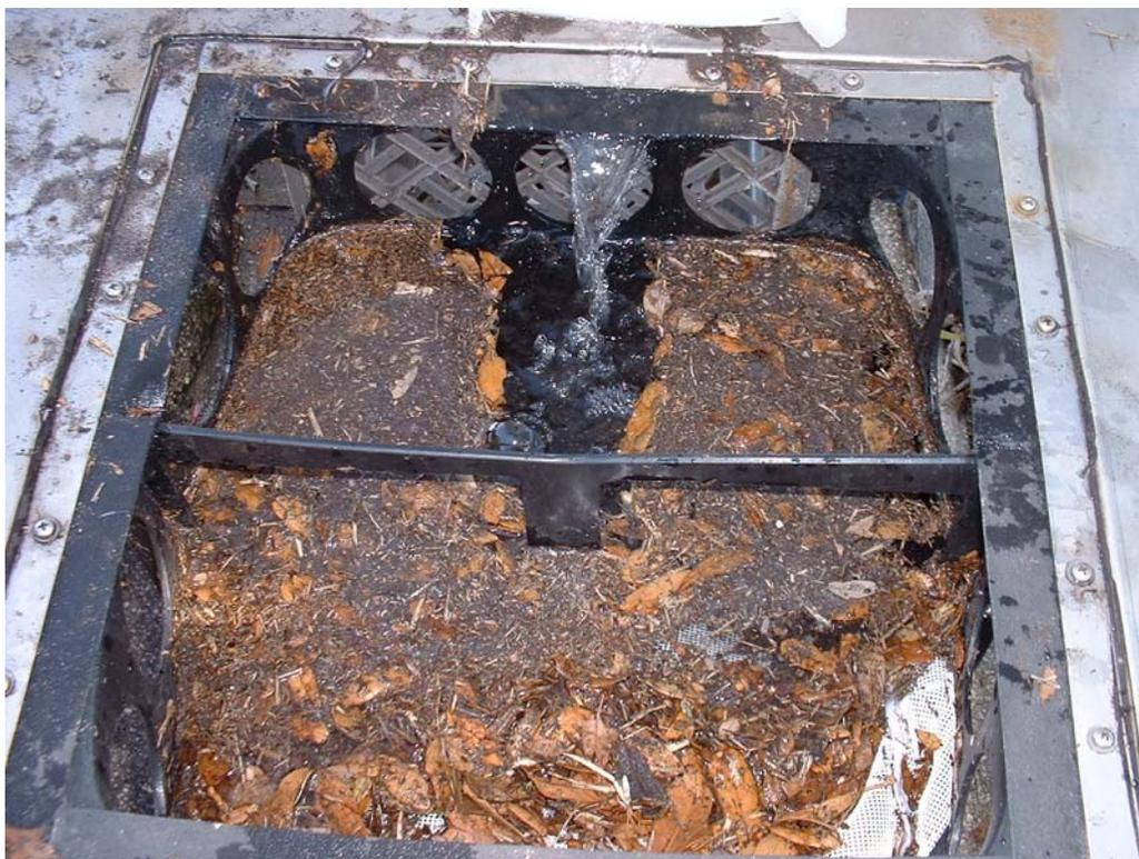
Figure 4-24. Accumulated Solids in the Hydro-Kleen Filter Unit.
