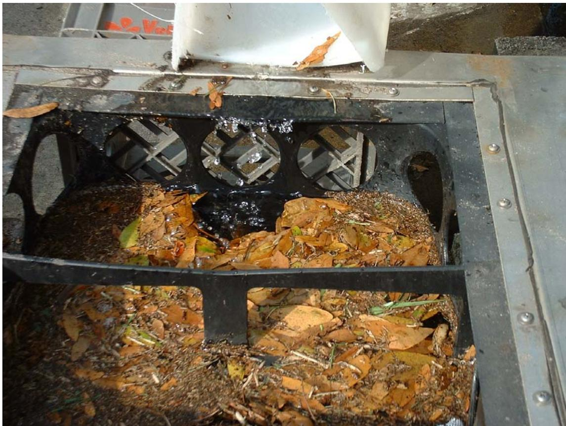
Figure 4-26. Loss of Leaves During Overflow of the Hydro-Kleen Filter Unit.
