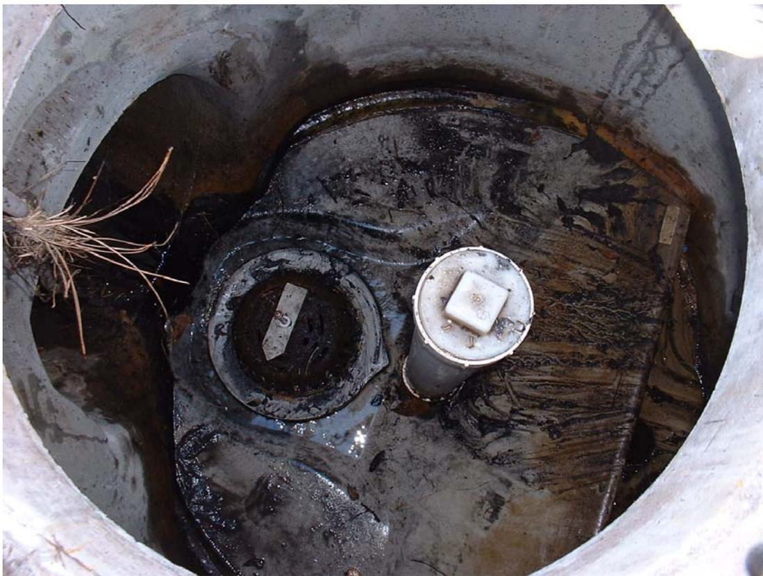
Figure 4-4. Stormsewer Inflow Bypassing the Stormceptor Unit Due to a Clogged Trash Grate.
