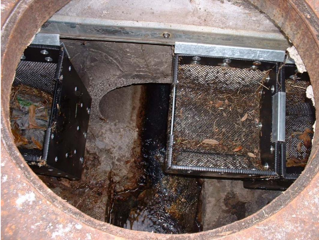
Figure 2-5. Ultra-Urban Filters Installed in Curb Inlet Structure.
