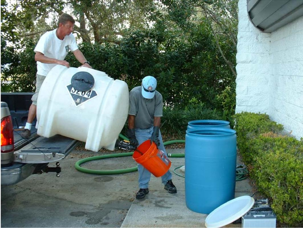
Figure 3-5. Stormceptor Sump Solids Transferred to 50-Gallon Barrels for Drying.
