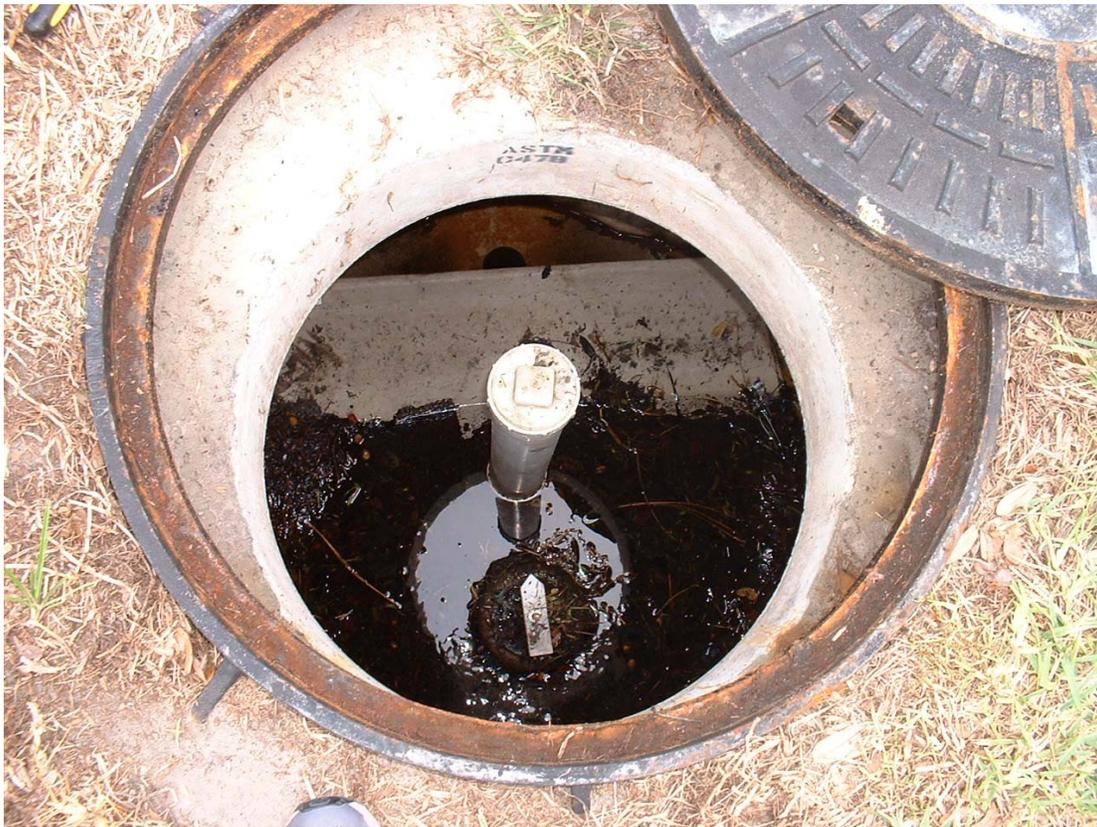
Figure 2-2. Photograph of the Stormceptor Unit Beneath the Manhole Cover.
