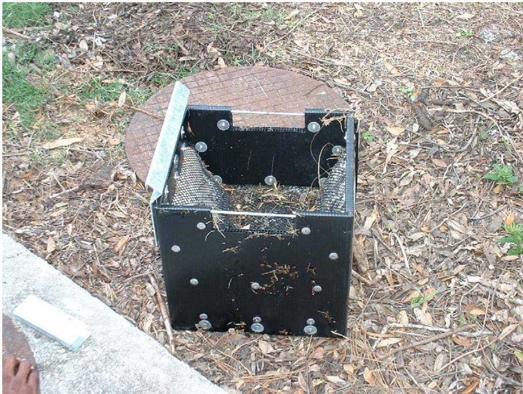
Figure 2-4. Ultra-Urban Filter Unit from the City of Palm Bay Installation.
