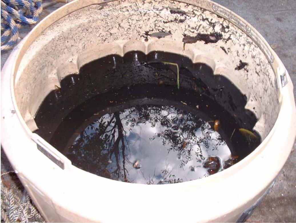
Figure 4-10. Sample of Solids Removed from Stormceptor Sump.
